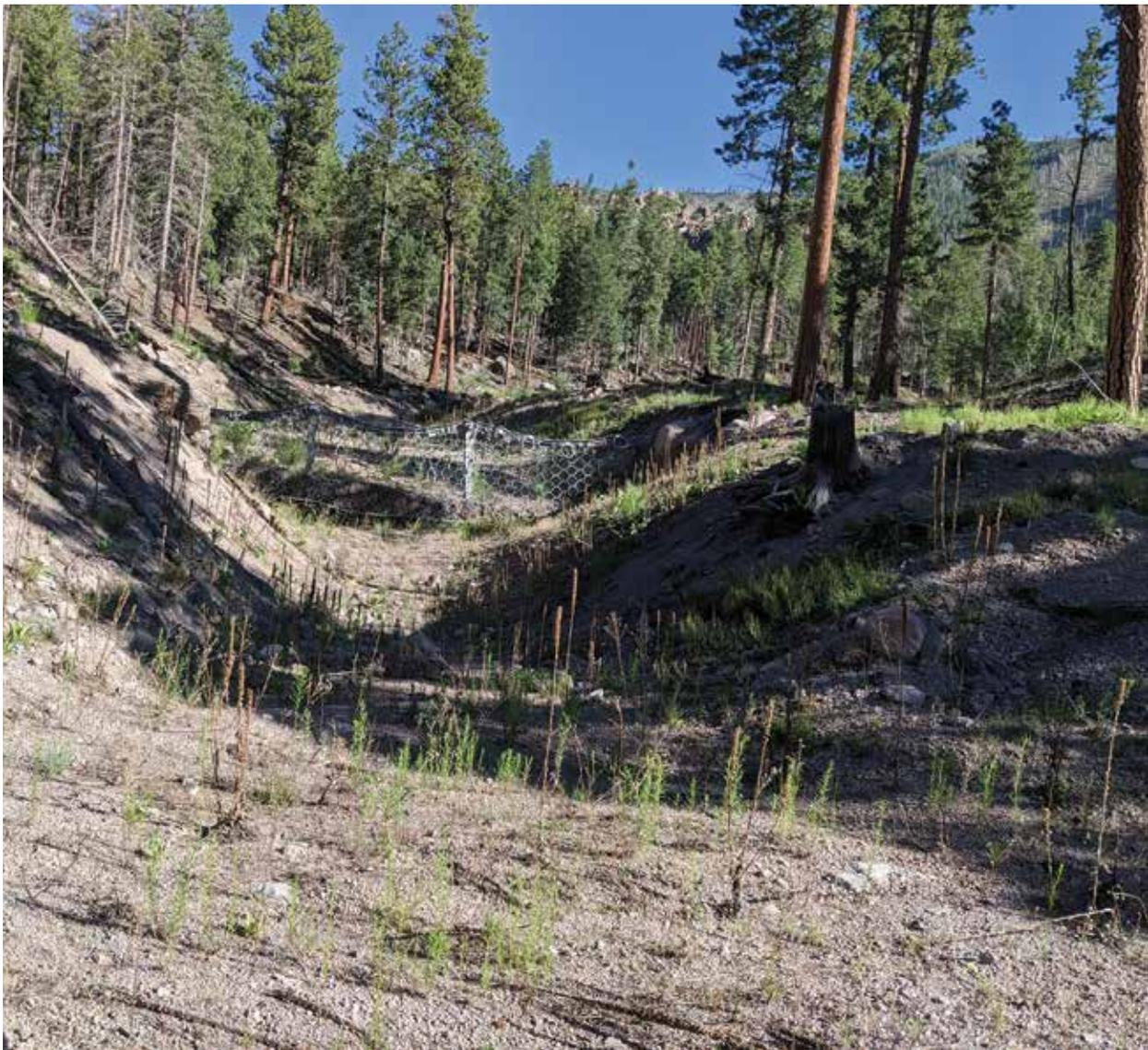
*A debris barrier gate, one of many structures placed to control erosion following the 2011 Las Conchas Fire, Santa Clara Pueblo. PHOTO CREDIT: JOHN SESSIONS*
